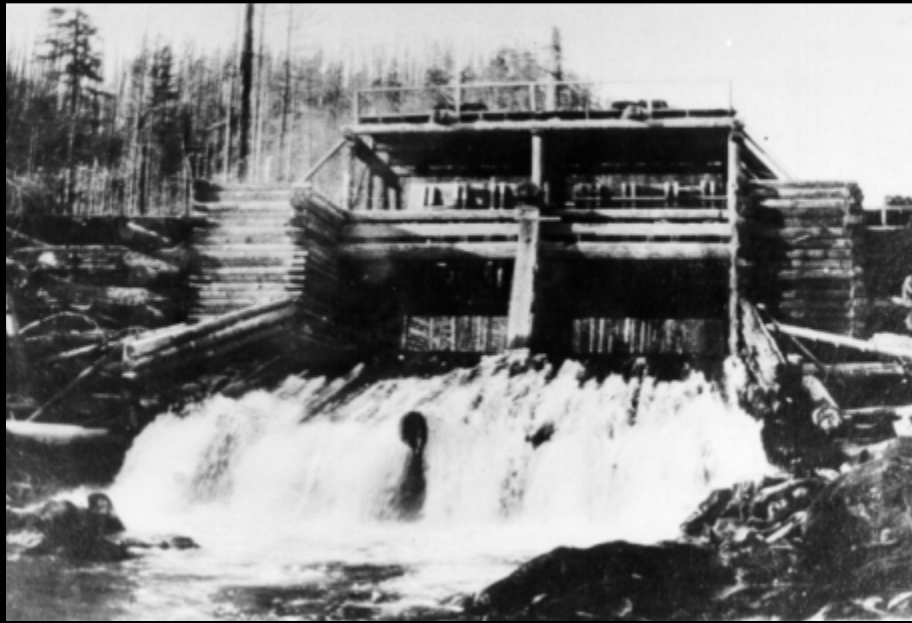
Splash Dam at the Hemlock Site—1902
