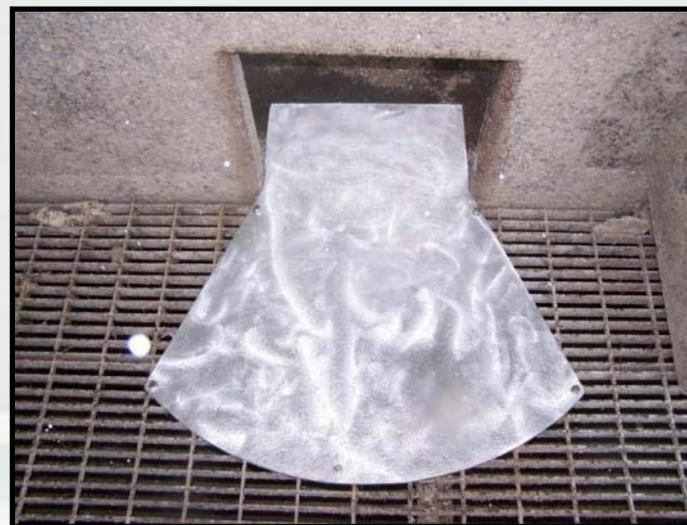
Diffuser plating at weir orifices
