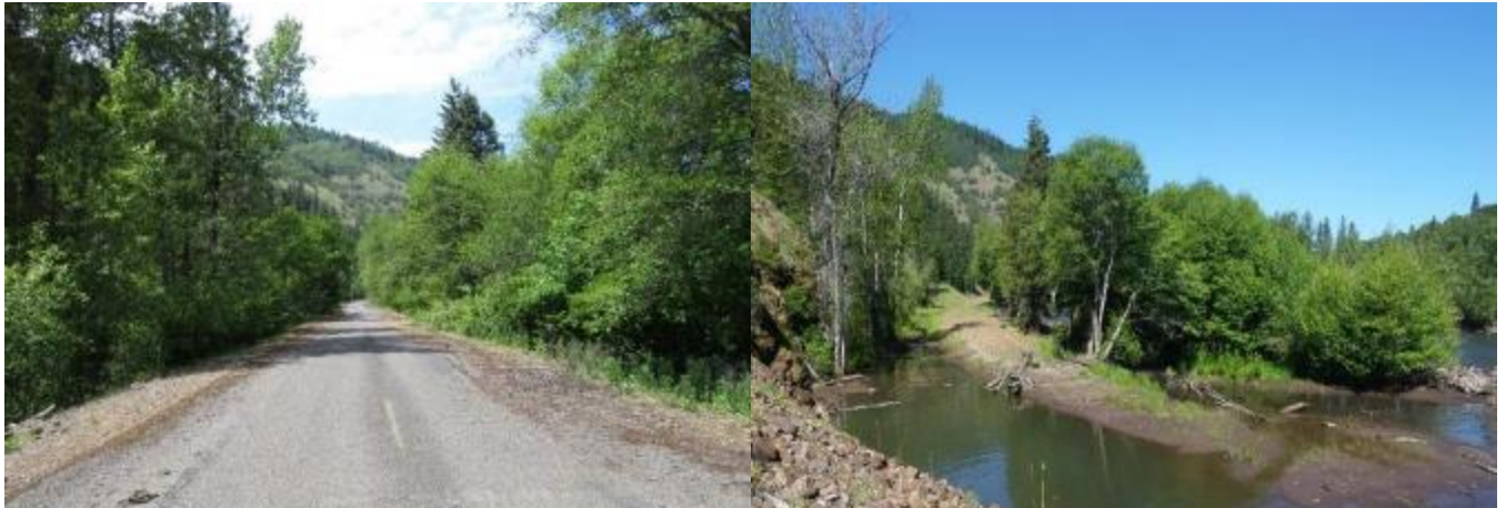
Figure 4. Haul Road segment 3.56 before (5/9/2012) and after (5/12/2016) treatment.
