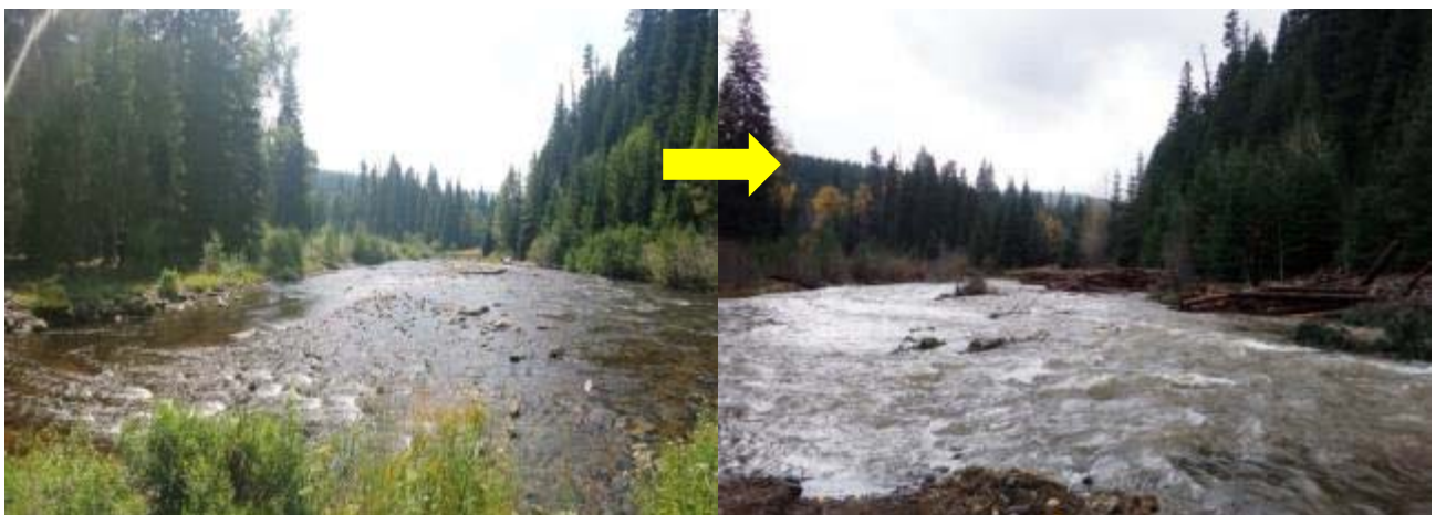
Figure 7. Pre- (left) and post-project (right) photos of constructed log jams along the right bank of the Klickitat River adjacent to 255 road.
