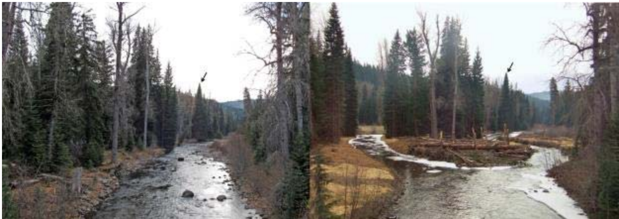
Figure 5. Pre- (left) and post-project (right) photos looking downstream from the 255 road crossing of the Klickitat River.
