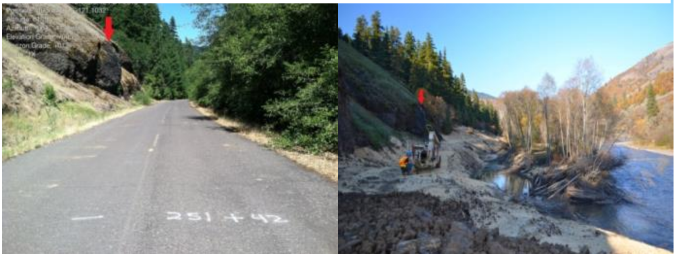
Figure 11. Klickitat River Floodplain Conservation and Restoration – Phase 4 pre (left) and after (right) removal of road prism, construction of channel and grading of floodplain.
