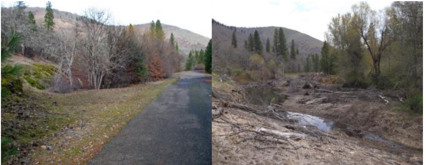
Figure 11. Klickitat River Floodplain Conservation and Restoration– Phase 3 pre (left) and after (right) removal of road prism, construction of channel and grading of floodplain.
