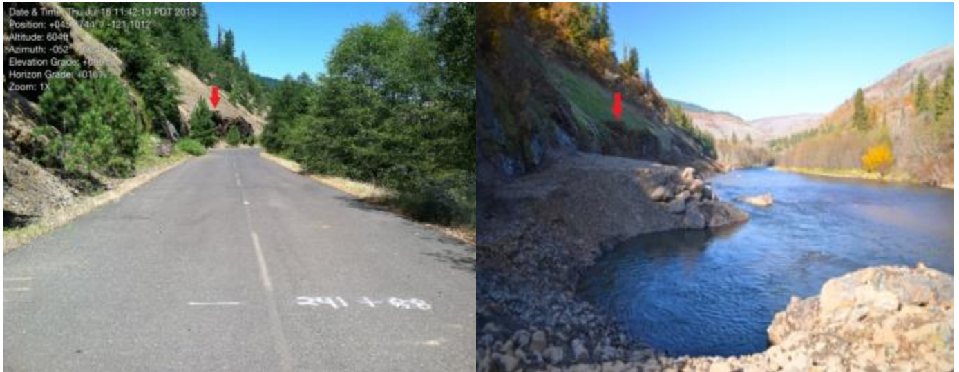
Figure 12. Klickitat River Floodplain Conservation and Restoration– Phase 4 pre (left) and after (right) removal of road prism and exposure of bedrock outcrop.
