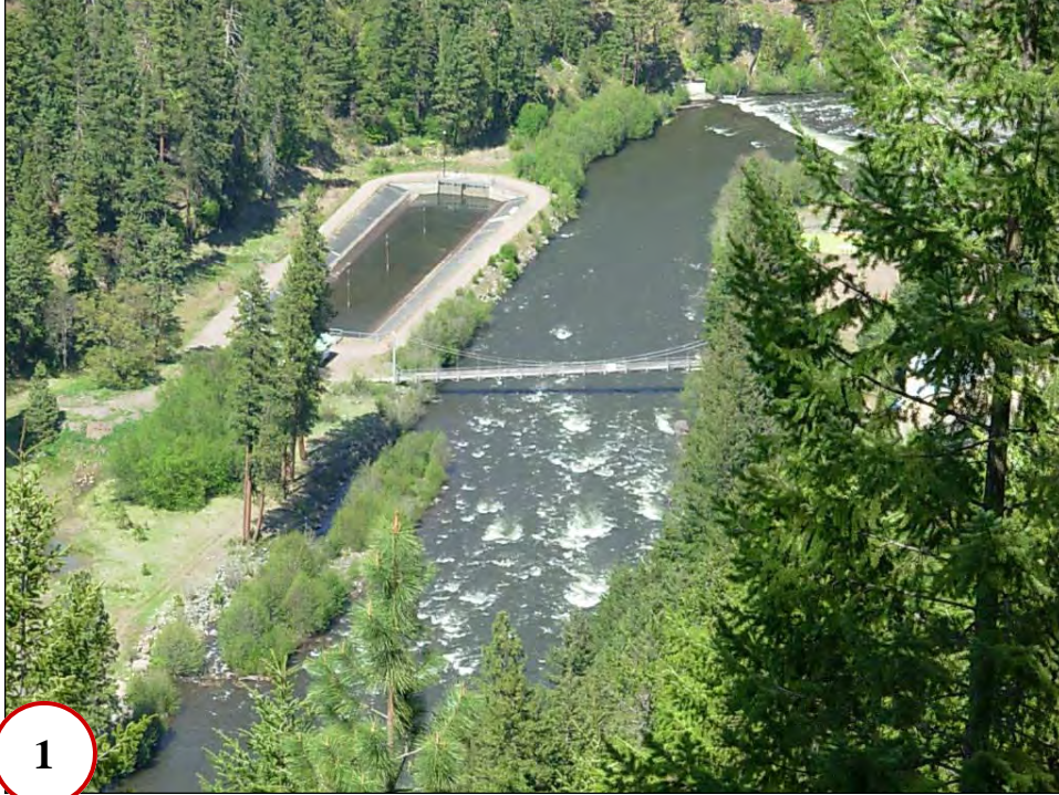
Klickitat River at Klickitat Hatchery looking downstream. Note existing suspension bridge at center and existing concrete sill visible at top of photo.
