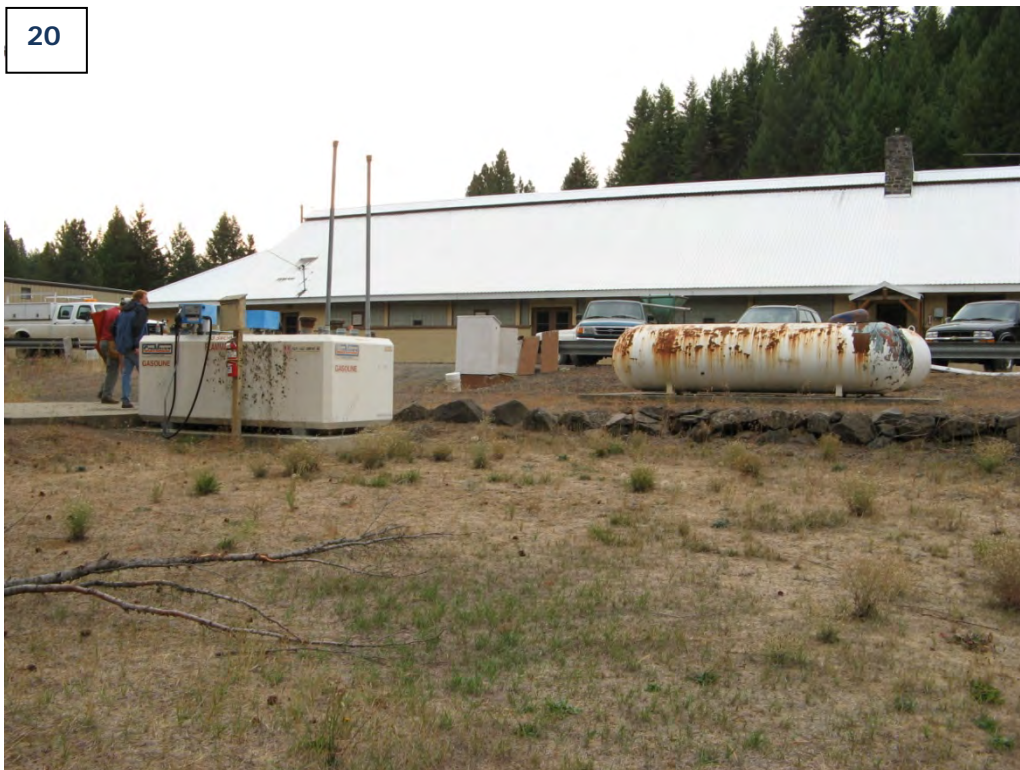
Propane Storage & Hatchery Building
