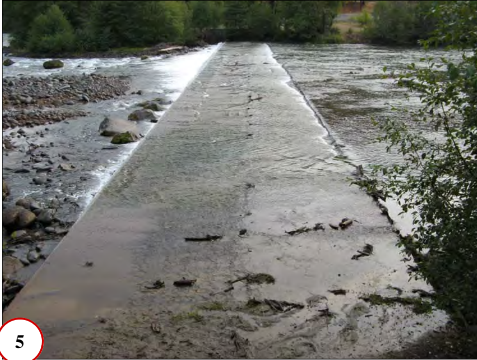
View of existing concrete sill from Klickitat River left bank.
