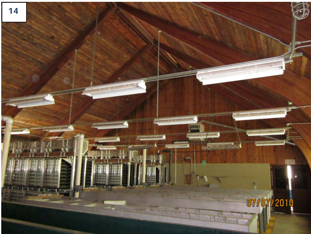
Hatchery Building Interior
