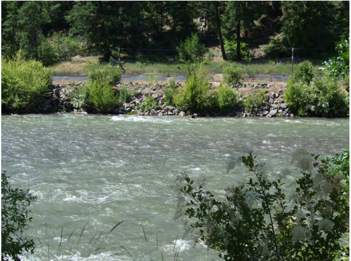
Plate 1b: looking across river from right bank, showing armoring on left bank.
