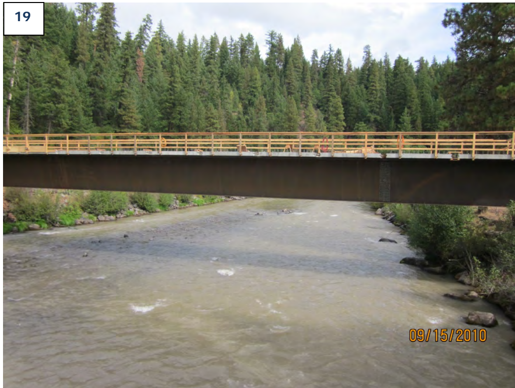
Bridge & Water Supply Lines
