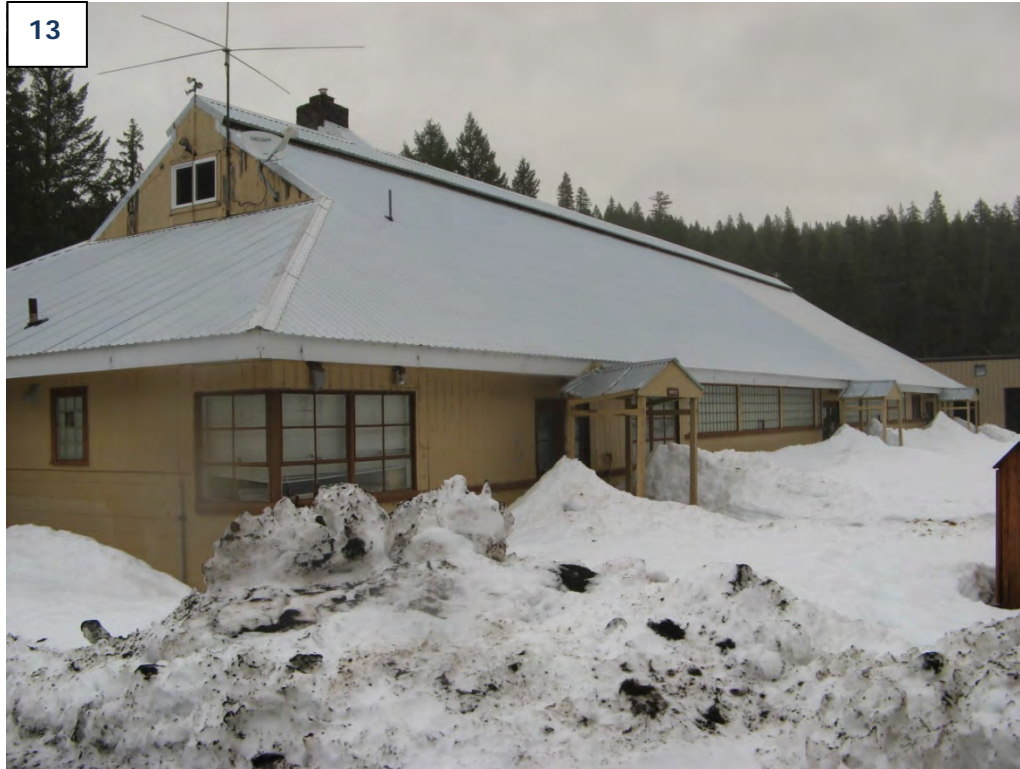
Hatchery Building Exterior
