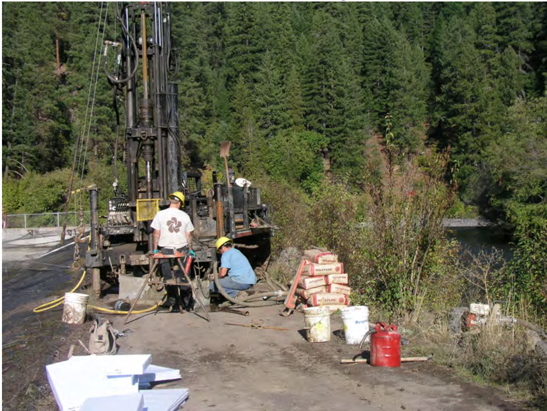
Plate 2b: BH-3 location on left bank dike by rearing pond 25.
