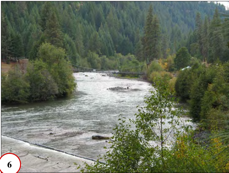
View looking upstream from existing concrete sill towards existing suspension bridge.
