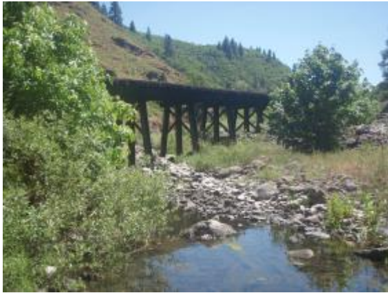
Unit 230 – Upstream view of train trestle
