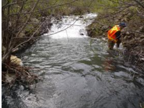
Unit 2 – Upstream view of plunge pool
